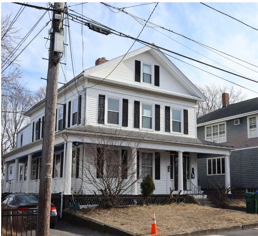
12 Maple Avenue Captain Redman House, 1845
