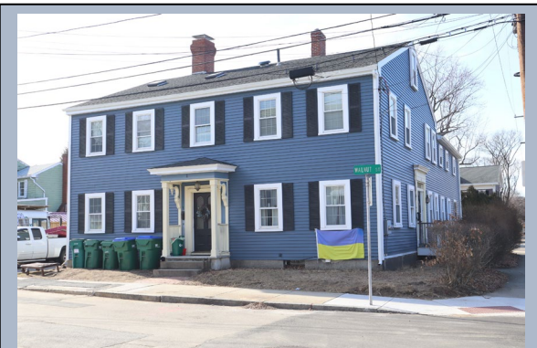
Bradbury Nichols House located at 1 Walnut Street
